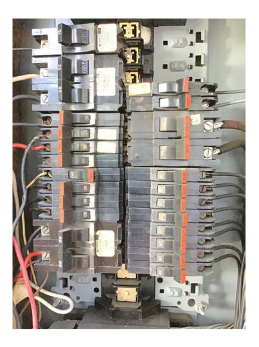
Reliance Electric Co., FPE's parent company, provided additional information that leads one to doubt how safe these panels are. Reliance Electric Co. has stated that FPE obtained the Underwriters Laboratory seal of approval for its Stab-Lok breakers "through the use of deceptive and improper practices."
