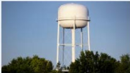
Elevated Tank/Booster Pump Station
