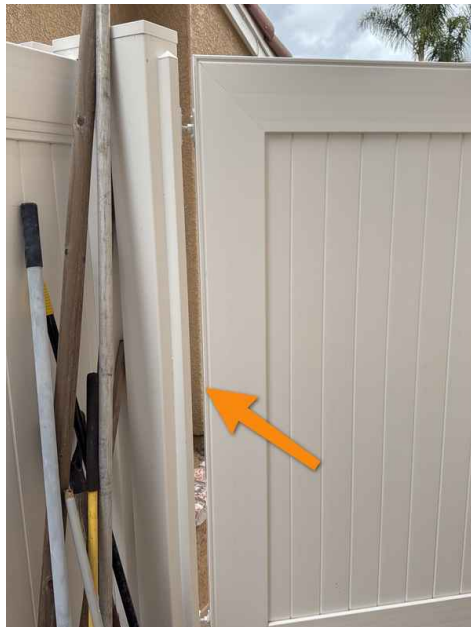
Self closing device needs adjustment
