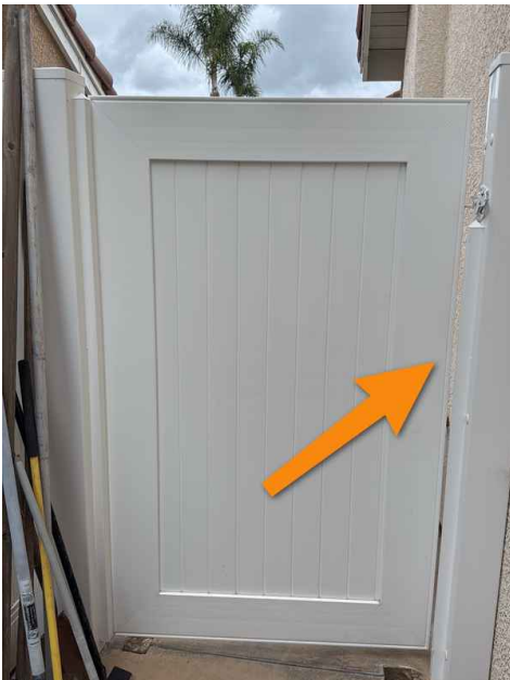
Self closing device needs adjustment
