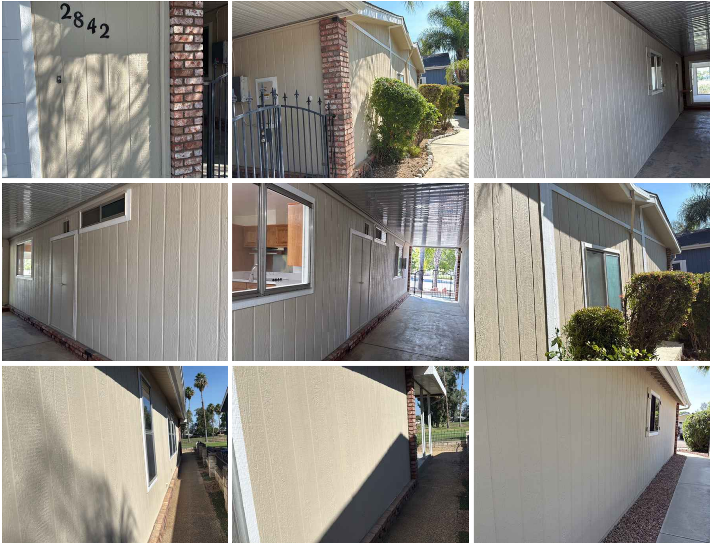
Siding, Flashing & Trim: Siding Material Engineered Wood, Brick
