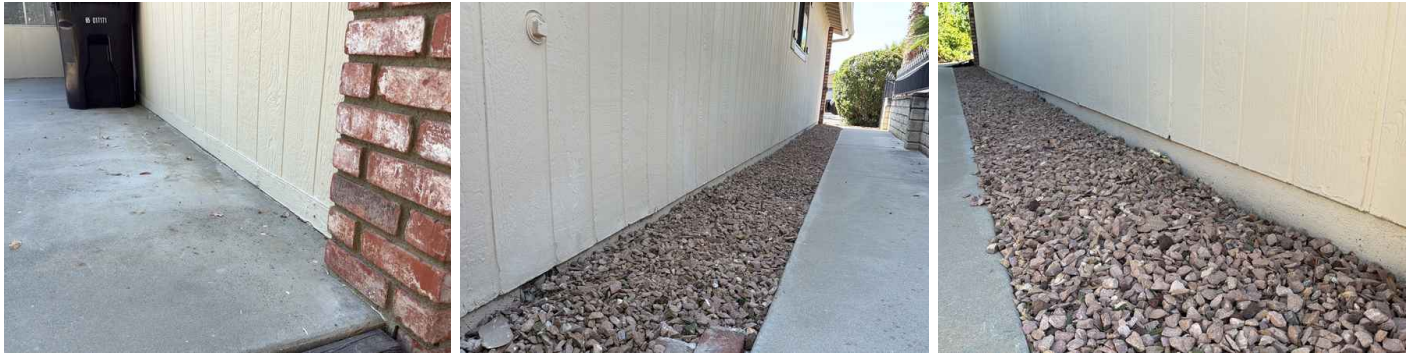
Siding, Flashing & Trim: Siding Material Engineered Wood, Brick
