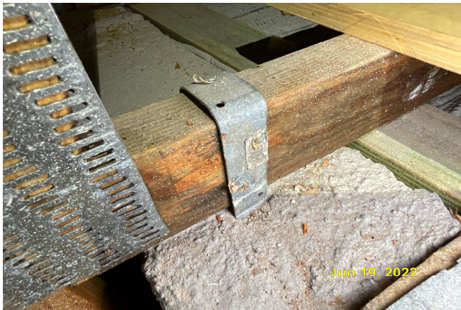
Single Wrap Strap (anchor side)
