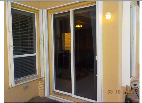
Glazed Door w/ Impact Acc Shutters
