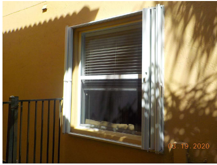
Window w/ Impact Accordion Shutters
