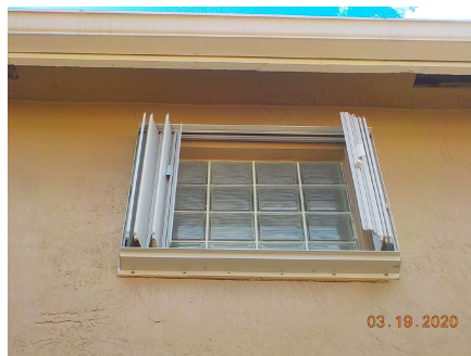
Glass Block w/ Impact Acc Shutters
