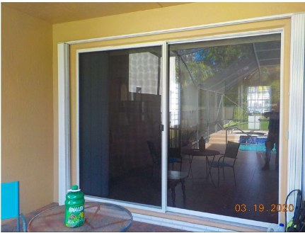
Glazed Door w/ Impact Acc Shutters
