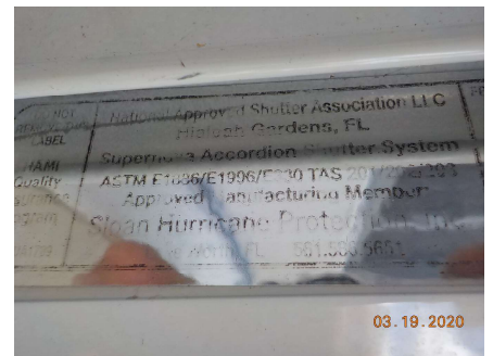
Accordion Shutter NOA (glass block)
