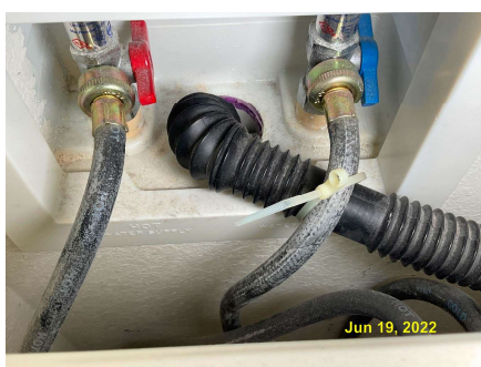
Washing Machine Connections
