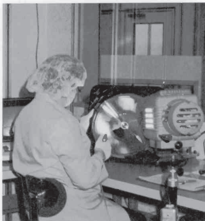
Fig. 6. Inspection station. The parts are inspected for defects using a grazing incidence light inspection, which highlights microscopic defects.
