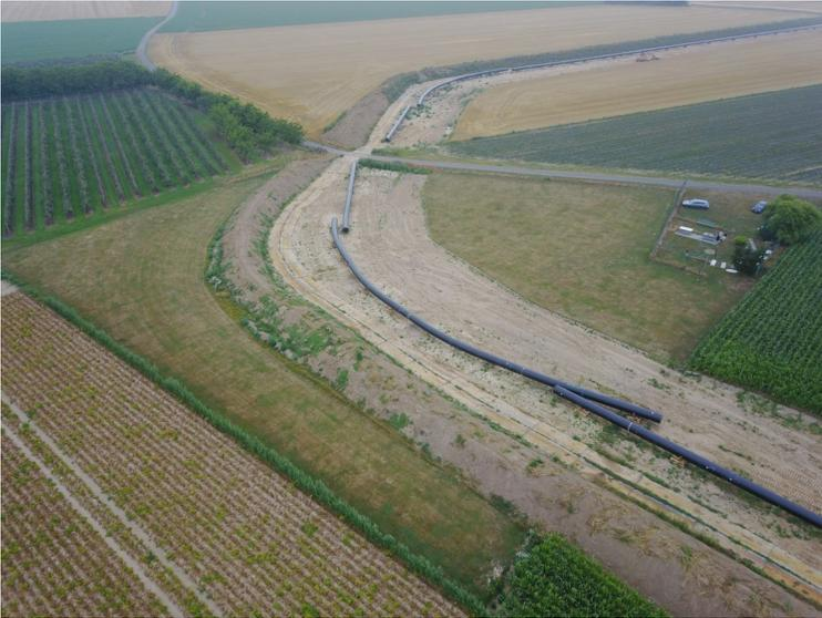
**The Zeelink Pipeline cutting across the field. The caged pit area is visible in upper right. A field boundary runs diagonally in lower left hand corner.**
