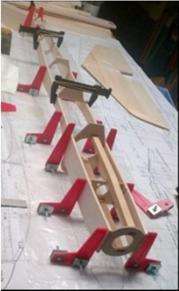
**Use of a magnetic building board in building the fuselage in space by Bernie Olson**
