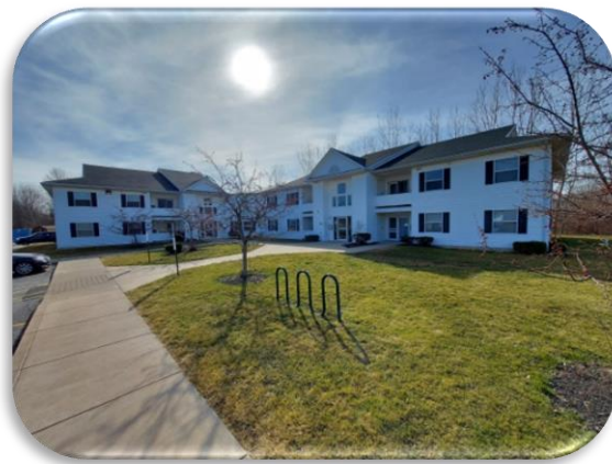
Wilson Villa Building 2 240 Autumnview Drive Wilson NY 14172 12 Two Bedroom Apartments
