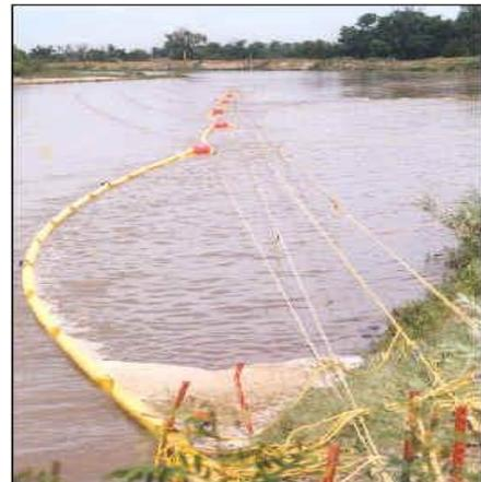
When using oil booms in flowing watercourses, two should be used – one immediately downstream of the other. This will allow the oil-saturated (upstream) boom to be removed without allowing the remaining oil to escape downstream. A replacement boom should then be located immediately downstream of the remaining boom.
