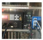
Wirelessly connects to NEMA street corner controllers. The portable traffic signal then assumes the standard function of the corner controller. The perfect solution for knockdowns.
