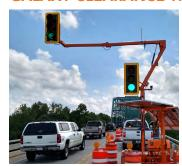
Detects slow moving vehicles in work zones and extends the red clearance interval in real time to ensure traffic safely clears the work zone before the interval expires.
