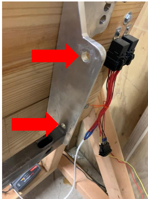
Figure 5 - Drilled Holes in Transom Bracket
