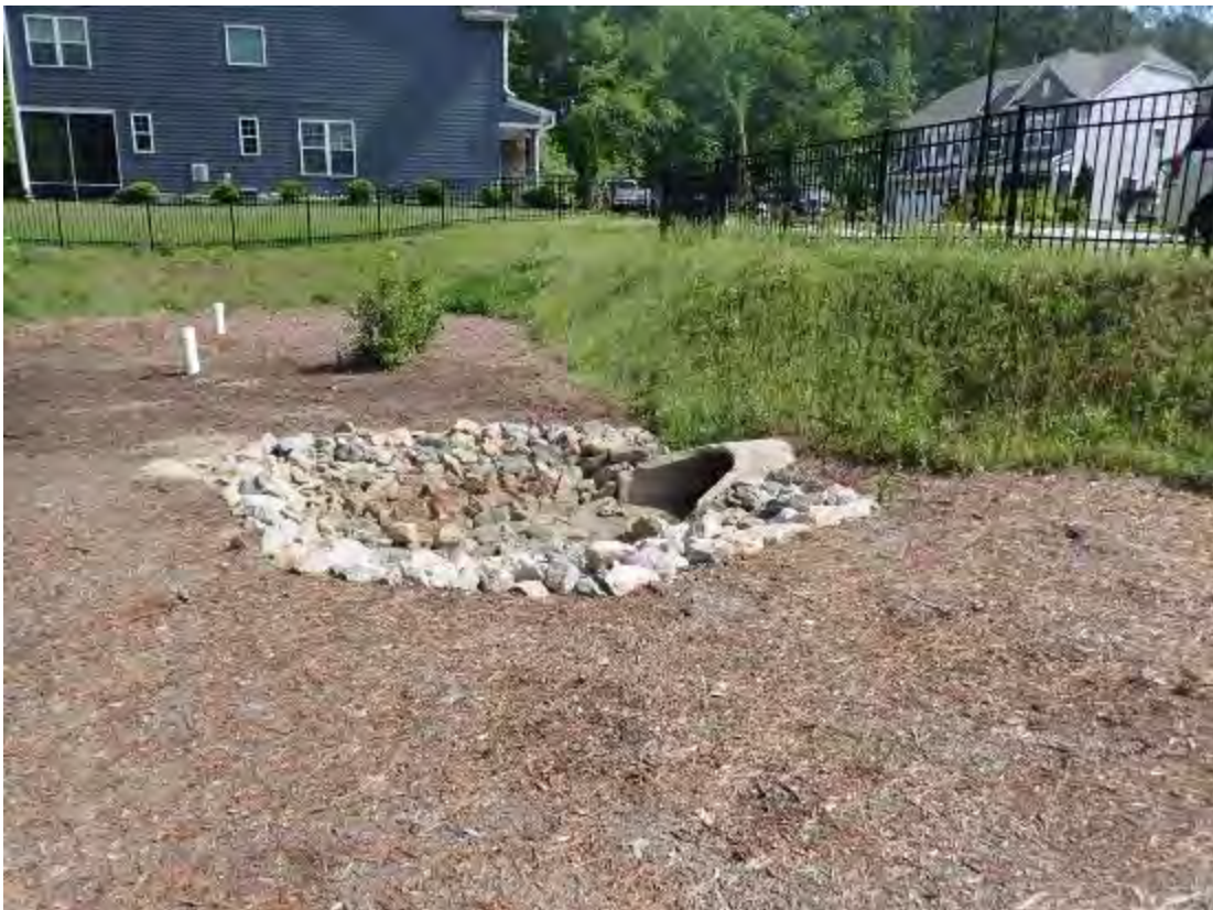
B: VIEW OF NORTH END OF CELL WITH INLET/FOREBAY
