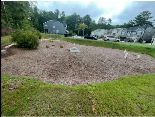
Overall view of BMP3
