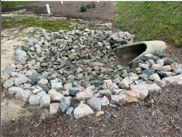
Inlet of BMP3
