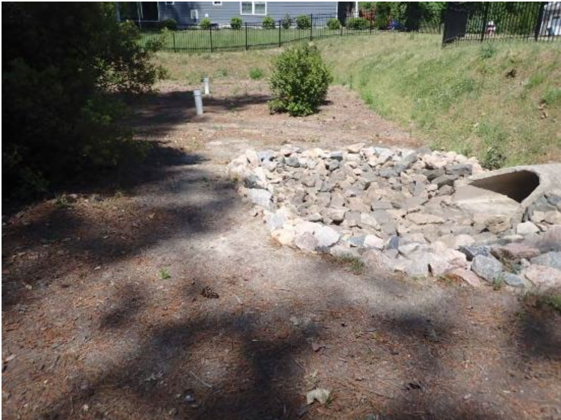
B: VIEW OF NORTH END OF CELL WITH INLET
