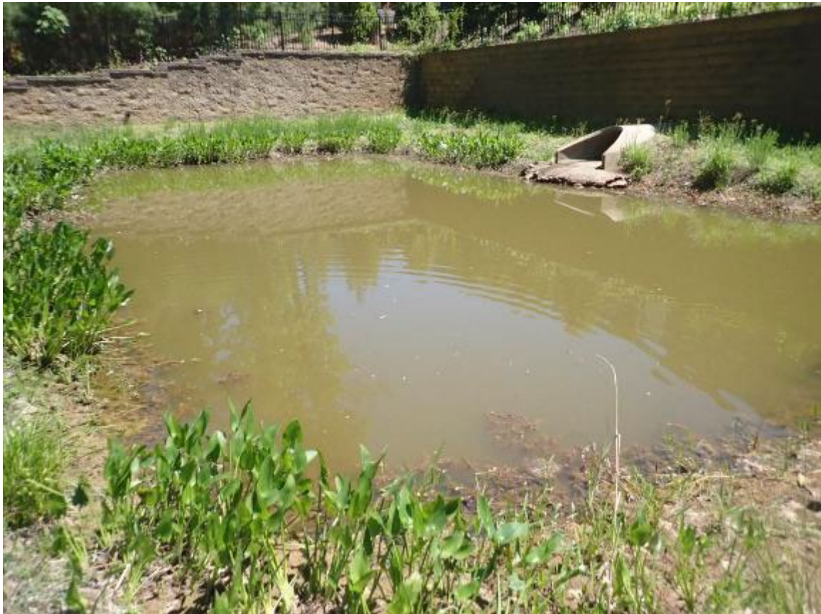
B: VIEWS OF FOREBAY AND INLET
