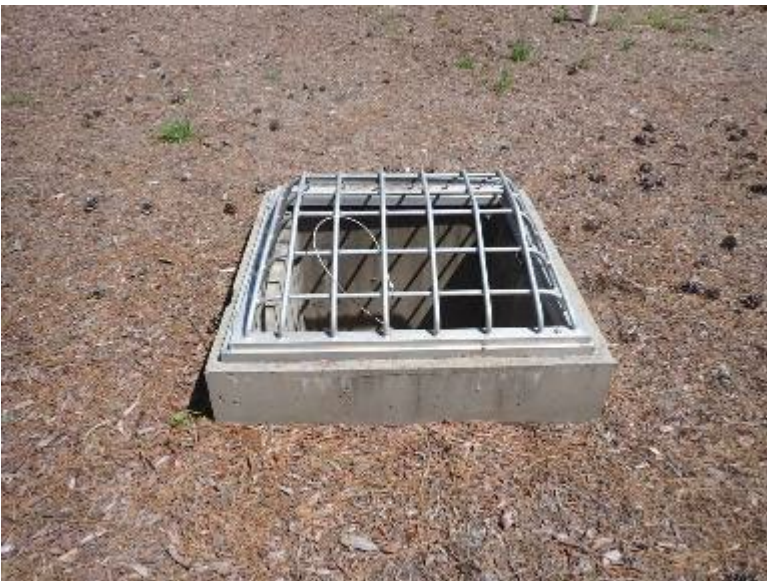
D: VIEW OF RISER OUTLET STRUCTURE EXTERIOR AND INTERIOR
