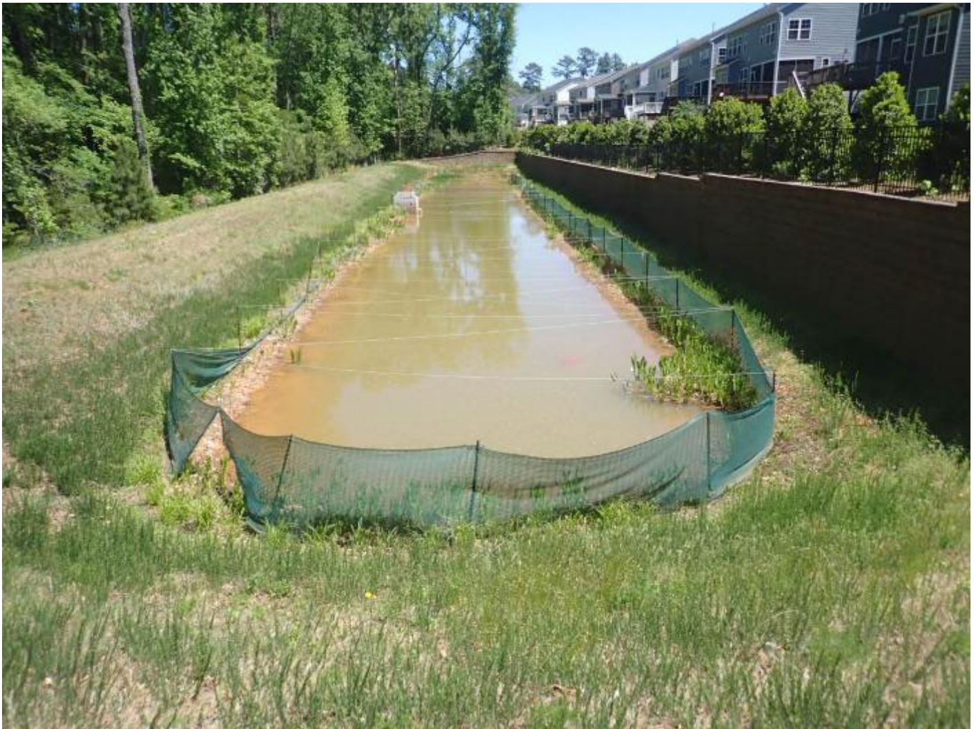
A: VIEW OF WET DETENTION POND
