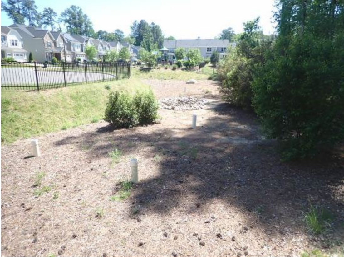
A: VIEW OF BIORETENTION
