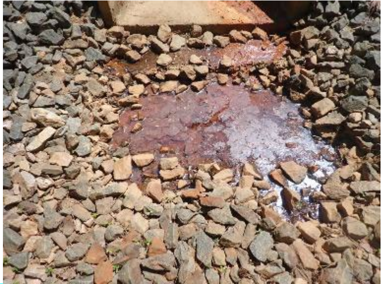
D: RESTORE STONE IN VOID FORMED AT OUTLET DISSIPATER: EITHER REPOSITION EXISTING SMALL STONE AND APPLY LIGHT CONCRETE SLURRY TO HOLD IN PLACE, OR SUPPLEMENT WITH CLASS B RIP-RAP
