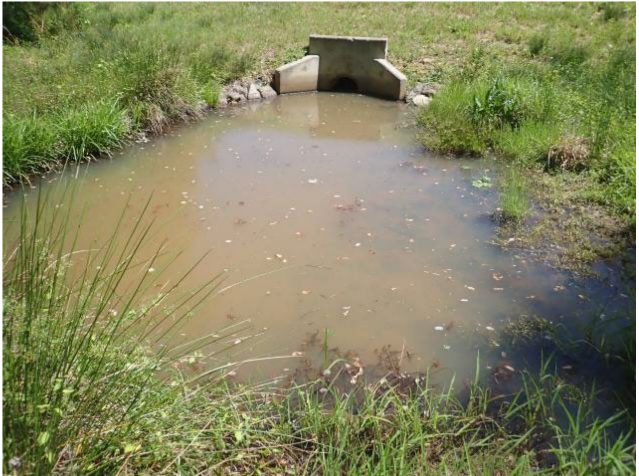
F: VIEW OF OUTLET DISCHARGE AREA
