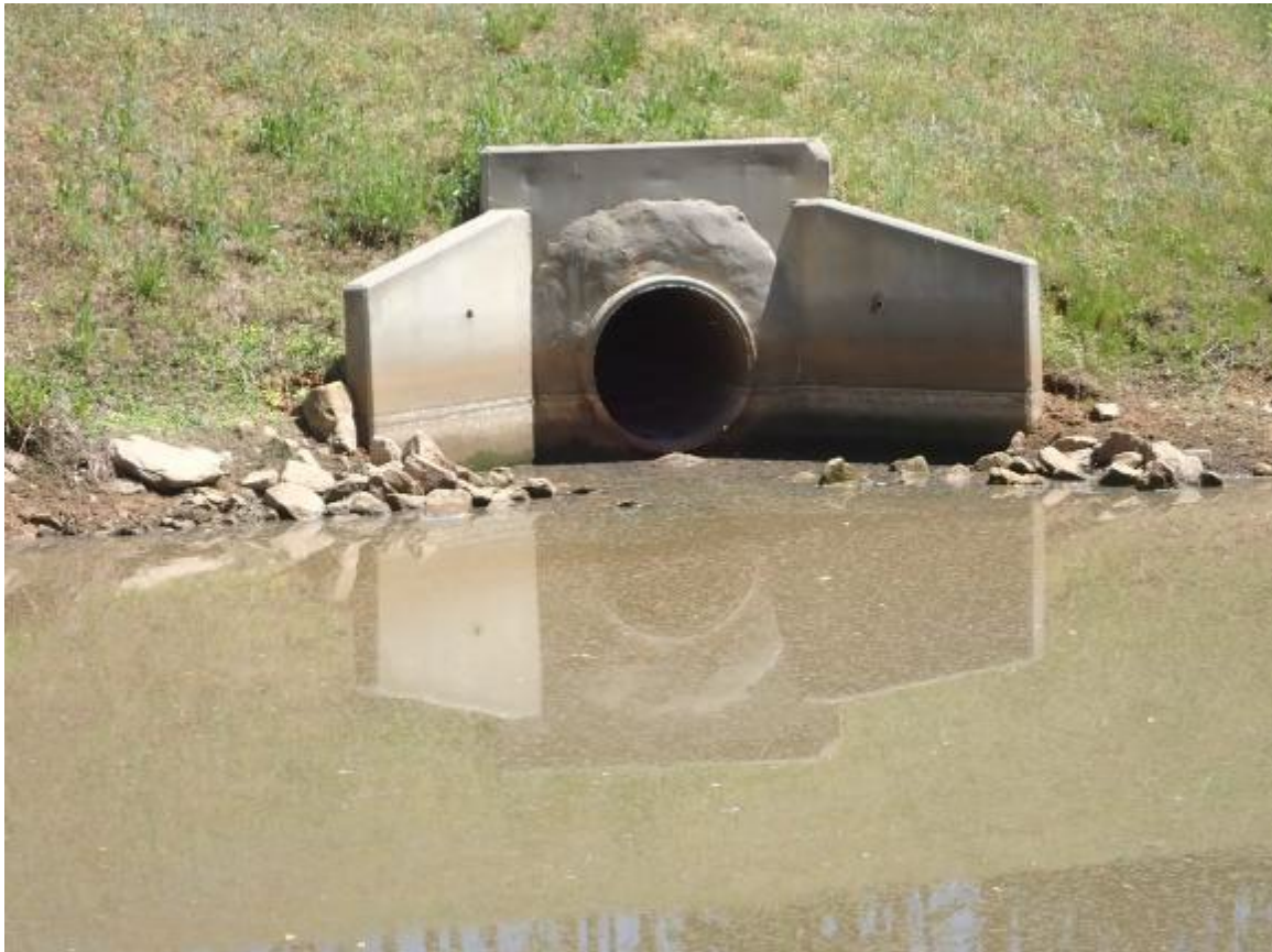
B: VIEW OF FOREBAY AND INLET
