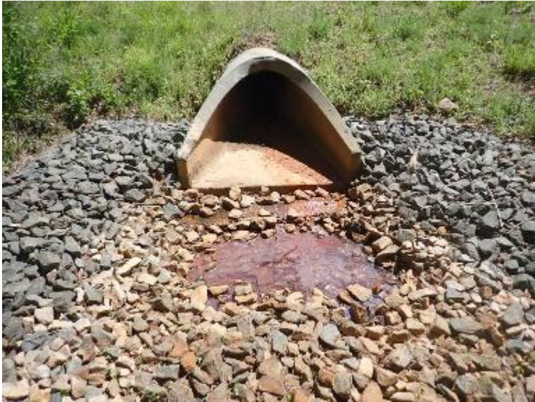
D: RESTORE STONE IN VOID FORMED AT OUTLET DISSIPATER: EITHER REPOSITION EXISTING SMALL STONE AND APPLY LIGHT CONCRETE SLURRY TO HOLD IN PLACE, OR SUPPLEMENT WITH CLASS B RIP-RAP
