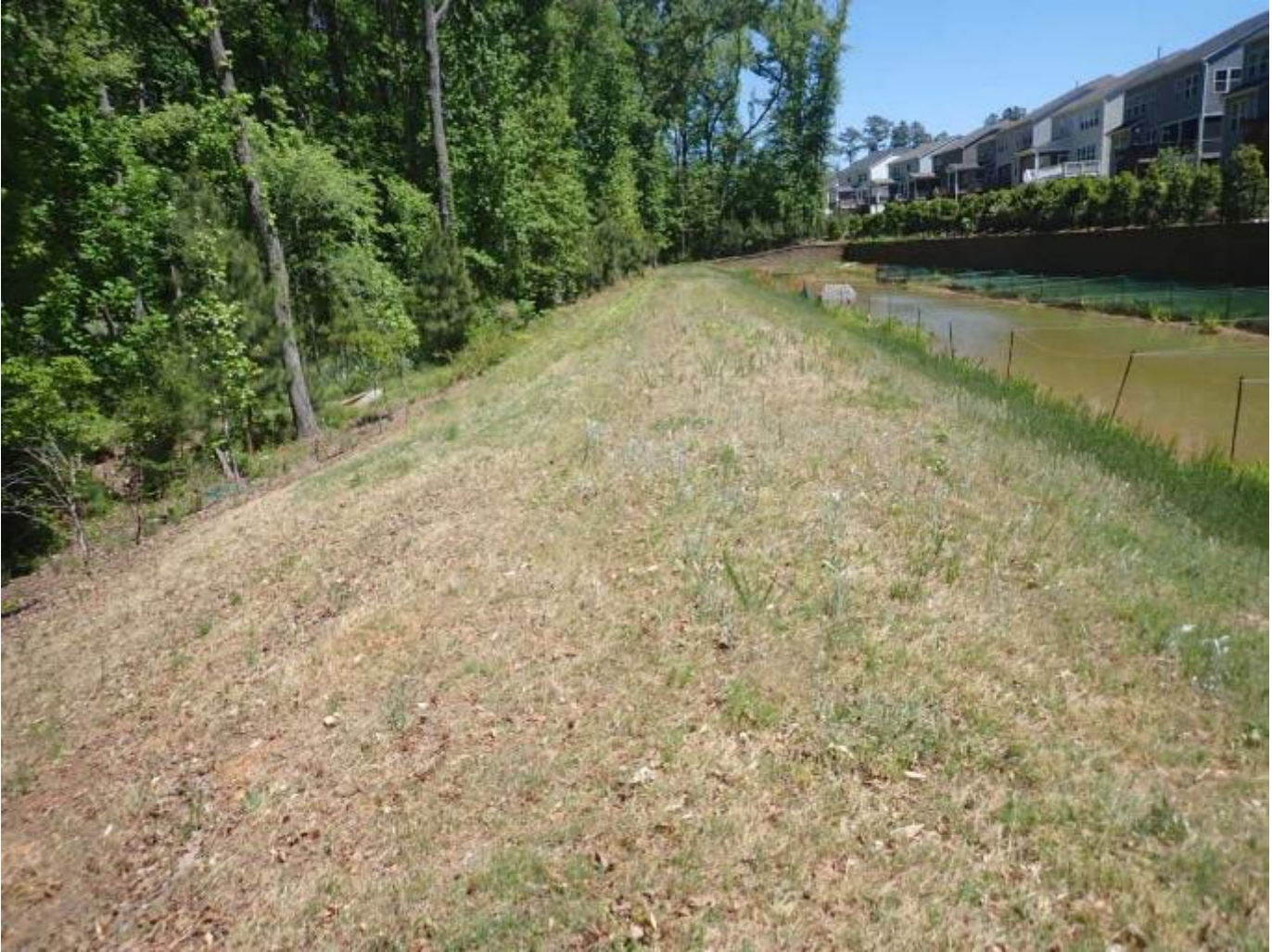
C: VIEW OF DAM EMBANKMENT
