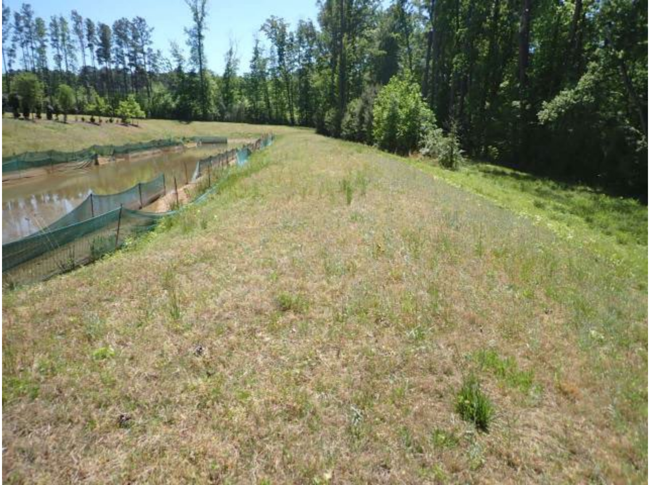
C: VIEW OF DAM EMBANKMENT
