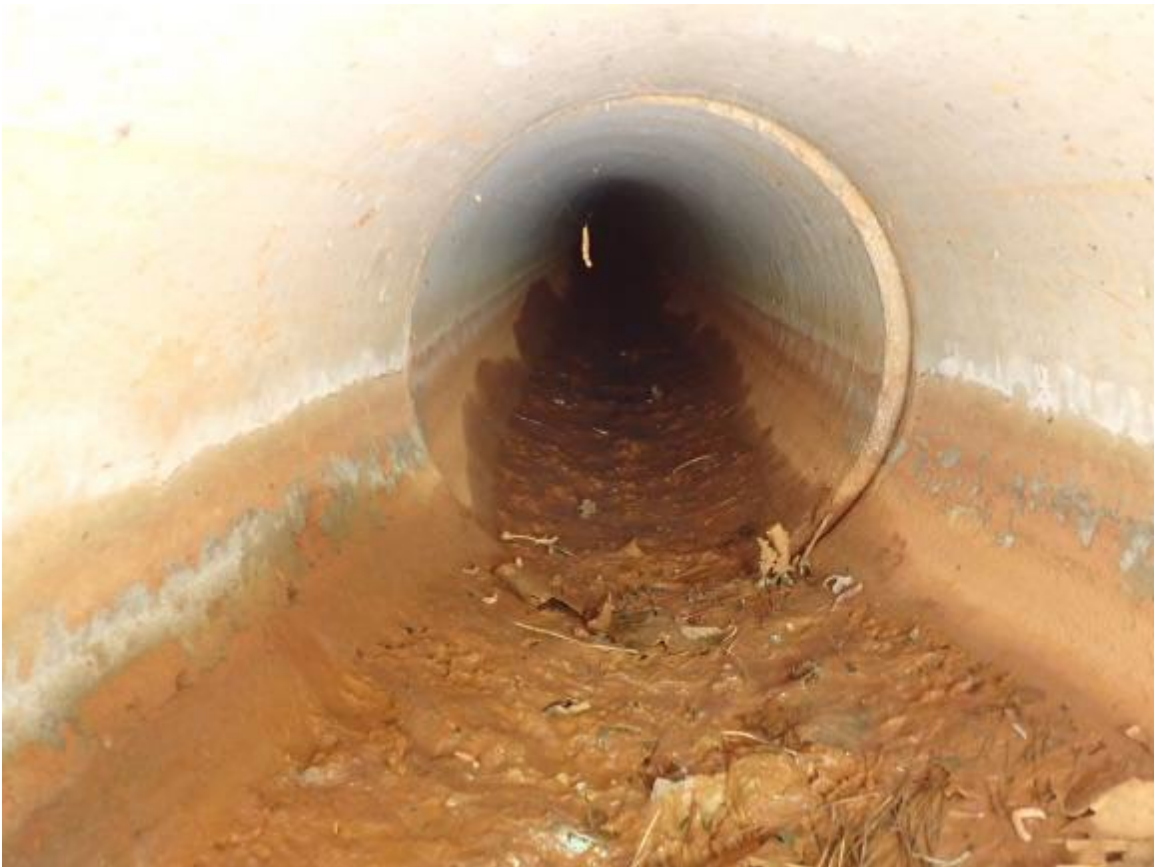
E: VIEWS OF OUTLET CONDUIT DISCHARGE
