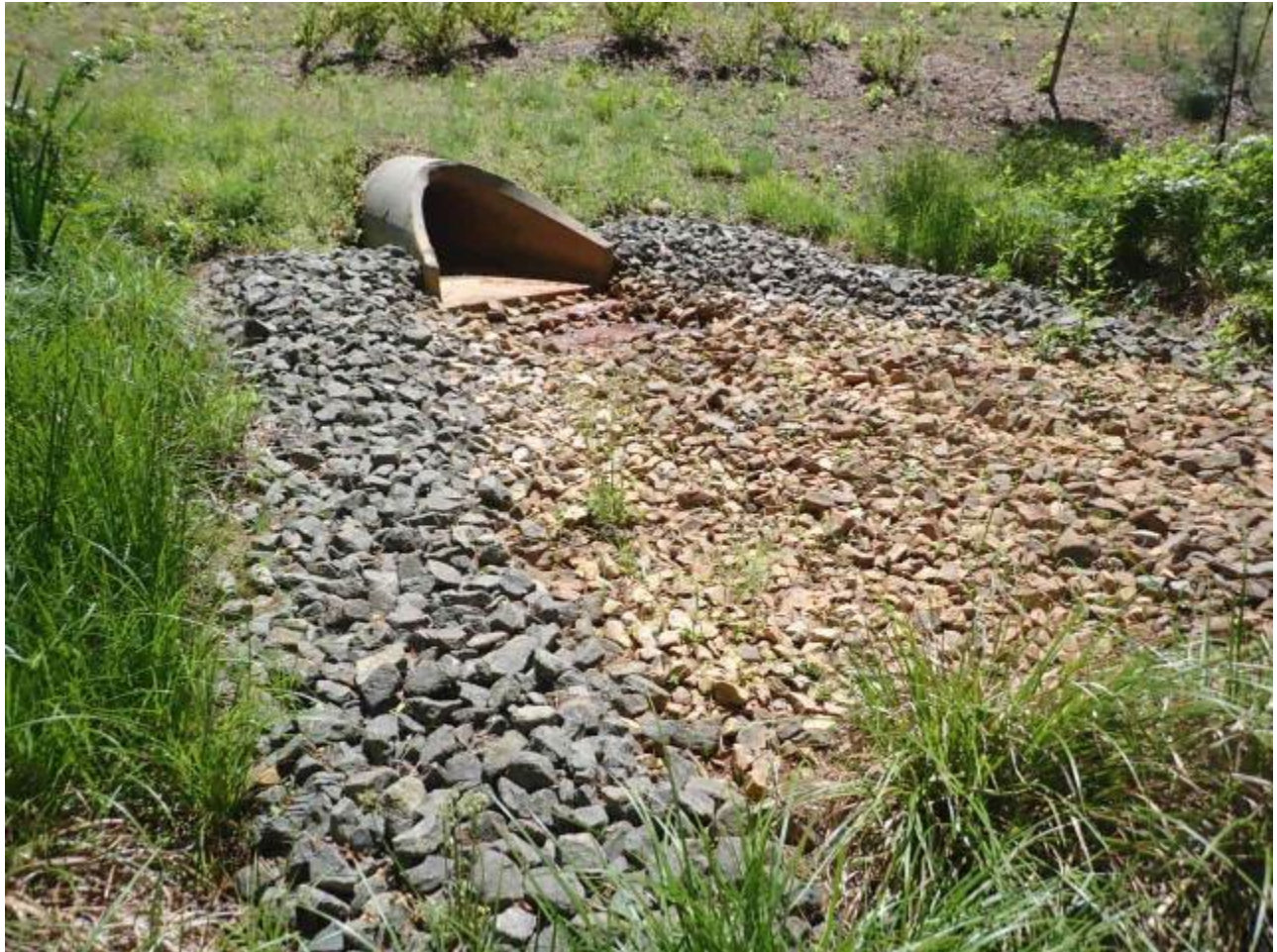
F: VIEW OF OUTLET DISCHARGE AREA
