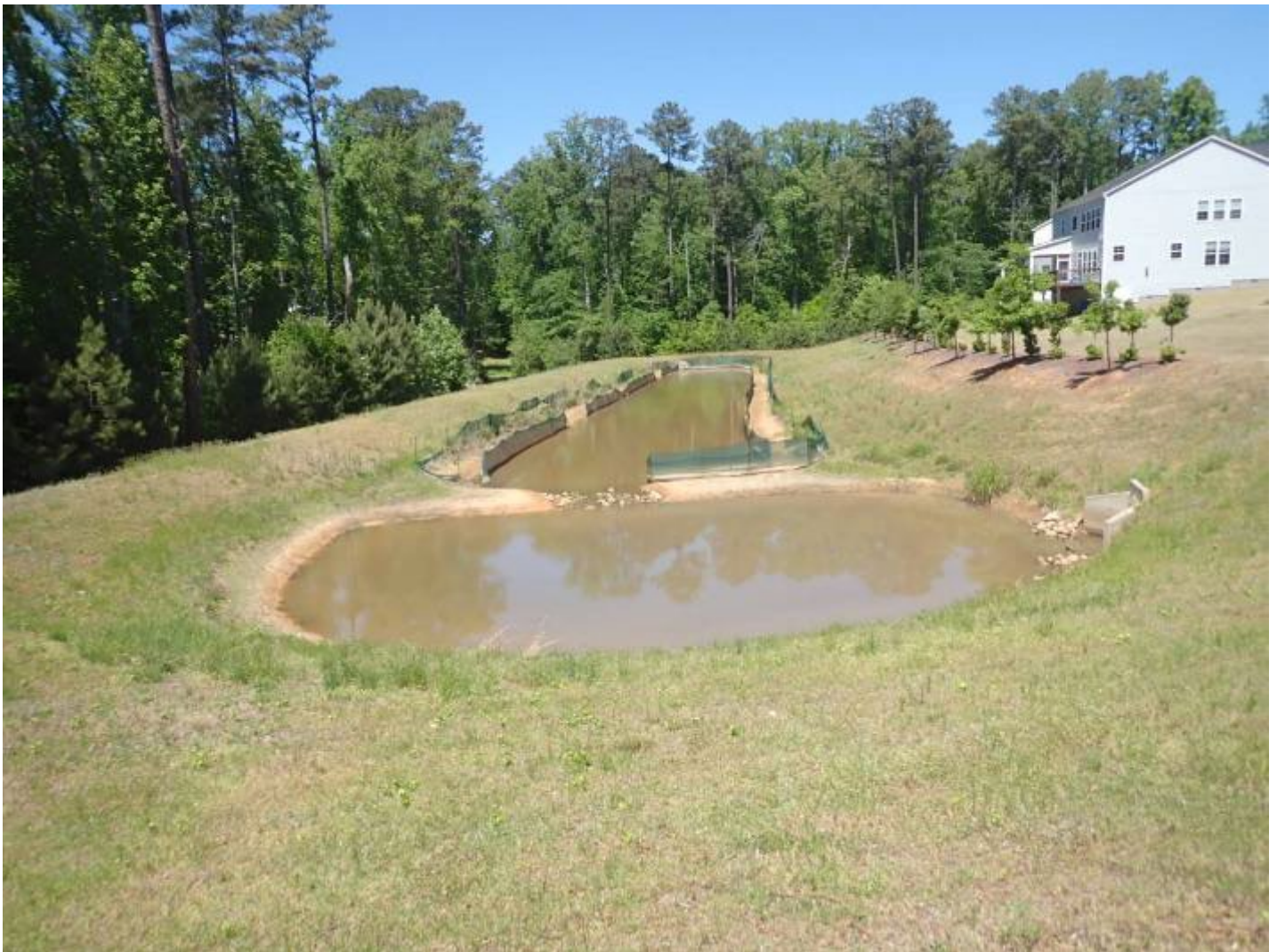
A: VIEW OF WET DETENTION POND
