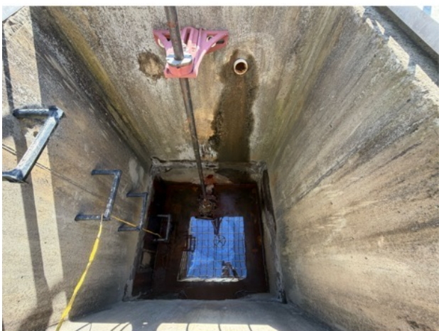
BMP 1 riser interior
