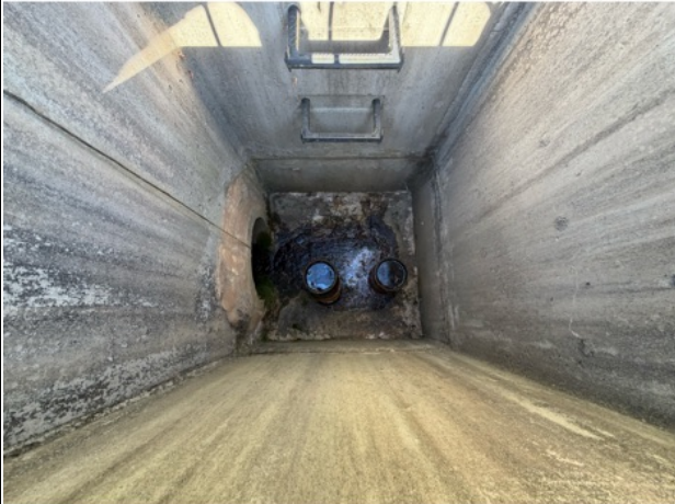
BMP 2 riser interior
