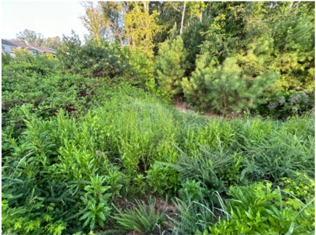
BMP3 Outlet easement overgrowth
