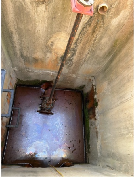
BMP1 Riser interior
