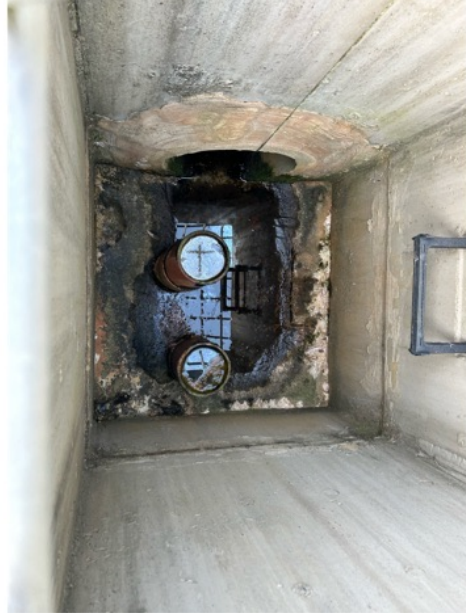
BMP3 Riser interior
