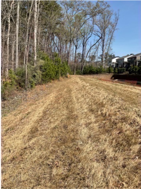
BMP2 back of dam
