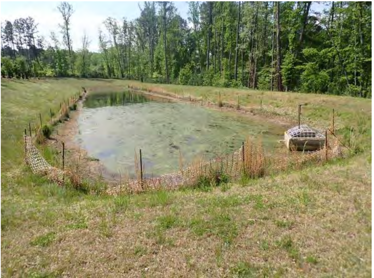
A: VIEW OF WET DETENTION POND
