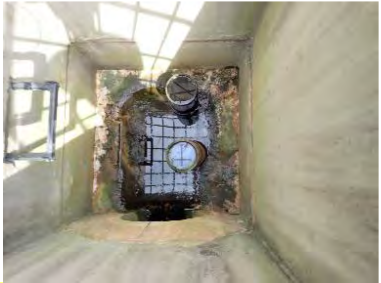
D: VIEW OF RISER OUTLET STRUCTURE EXTERIOR AND INTERIOR (FUNCTIONAL INTERNAL WATER STORAGE CONFIRMED)
