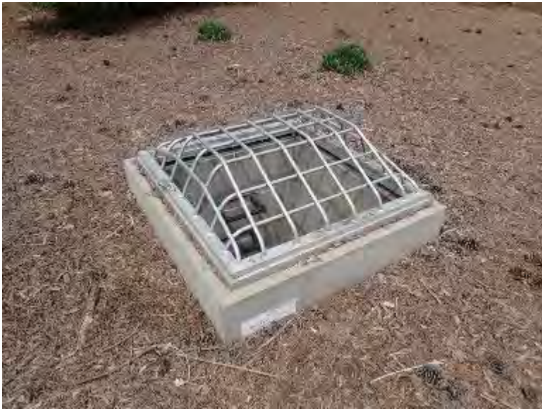
D: VIEW OF RISER OUTLET STRUCTURE EXTERIOR AND INTERIOR (FUNCTIONAL INTERNAL WATER STORAGE CONFIRMED)
