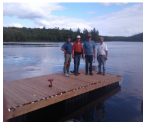
Some of the volunteers who built the new dock.
