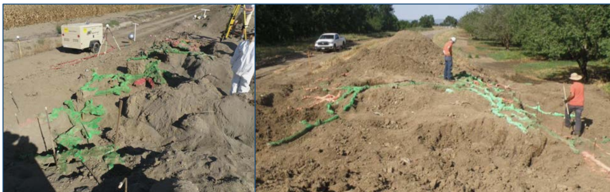
Figure 3. Colored Grout on Extensive Ground Squirrel Burrow Network
