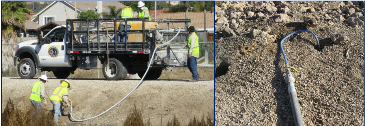
Figure 11. WPD Grout Machine at Levee with water Truck and Hose
