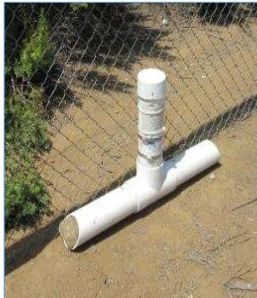
Figure 22. Vandalized Bait Station at Conejo Mountain Basin No. 1
