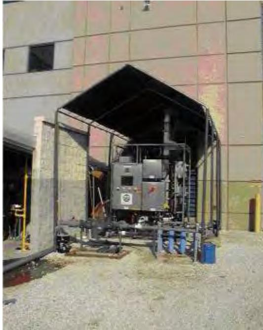
**Figure 3.14 Membrane B pilot unit as installed at the Tampa Bay Regional Water Treatment Plant**
