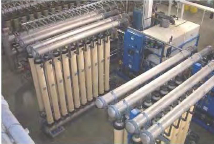
**Figure 3.33 Pall Microza MF skids as installed at Parsons, Kan.**
