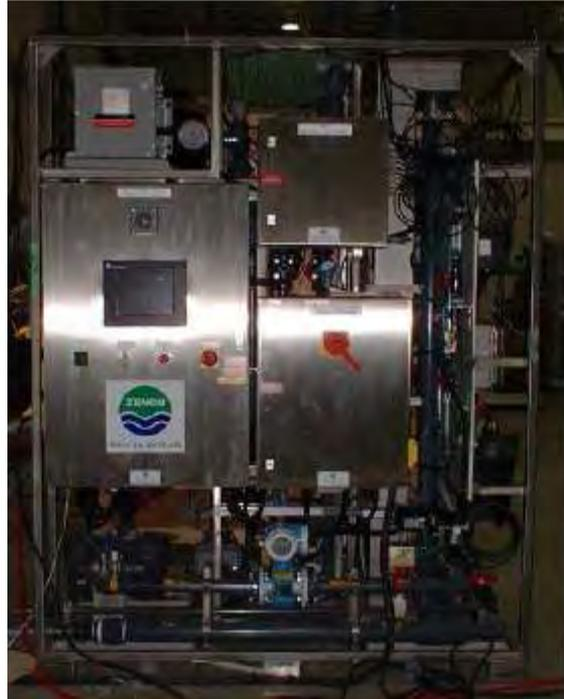
**Figure 3.30 Zenon ZeeWeed 1000 pilot system (Tuscaloosa) using Membrane B**
