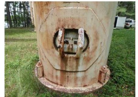
Shows riser manhole in very poor condition with heavy rusting.
