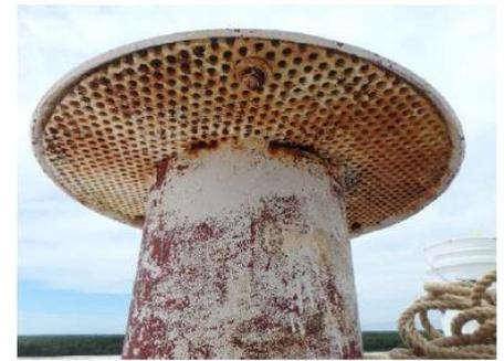
the perforated metal vent screen is in poor condition with medium rusting, and with heavy rust on the retention bolts.
