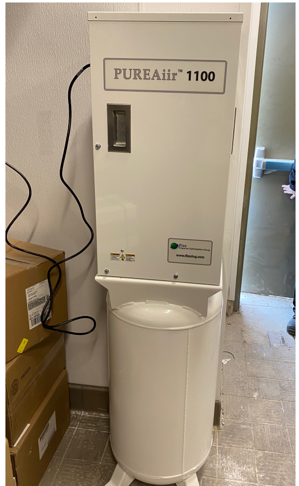
The PureAir and the storage tank can be remotely installed in separate locations.
