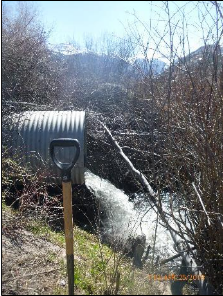
Photo 5. Wetland at culvert along Remine Creek.
