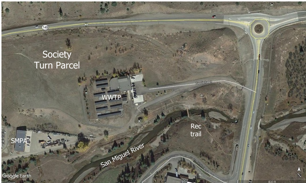
Photo 2. Aerial image of eastern portion of Society Turn Parcel. Note the location of the San Miguel River, nearby facilities, Highway 145 on the north and east, and part of a recreational trail and bridge. (This Google Earth image is from 10/12/15).
