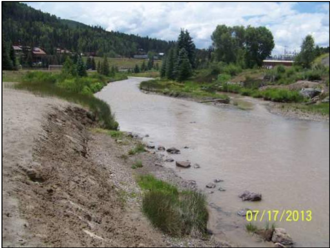
Photo 10. Narrow band of wetlands on north bank.
