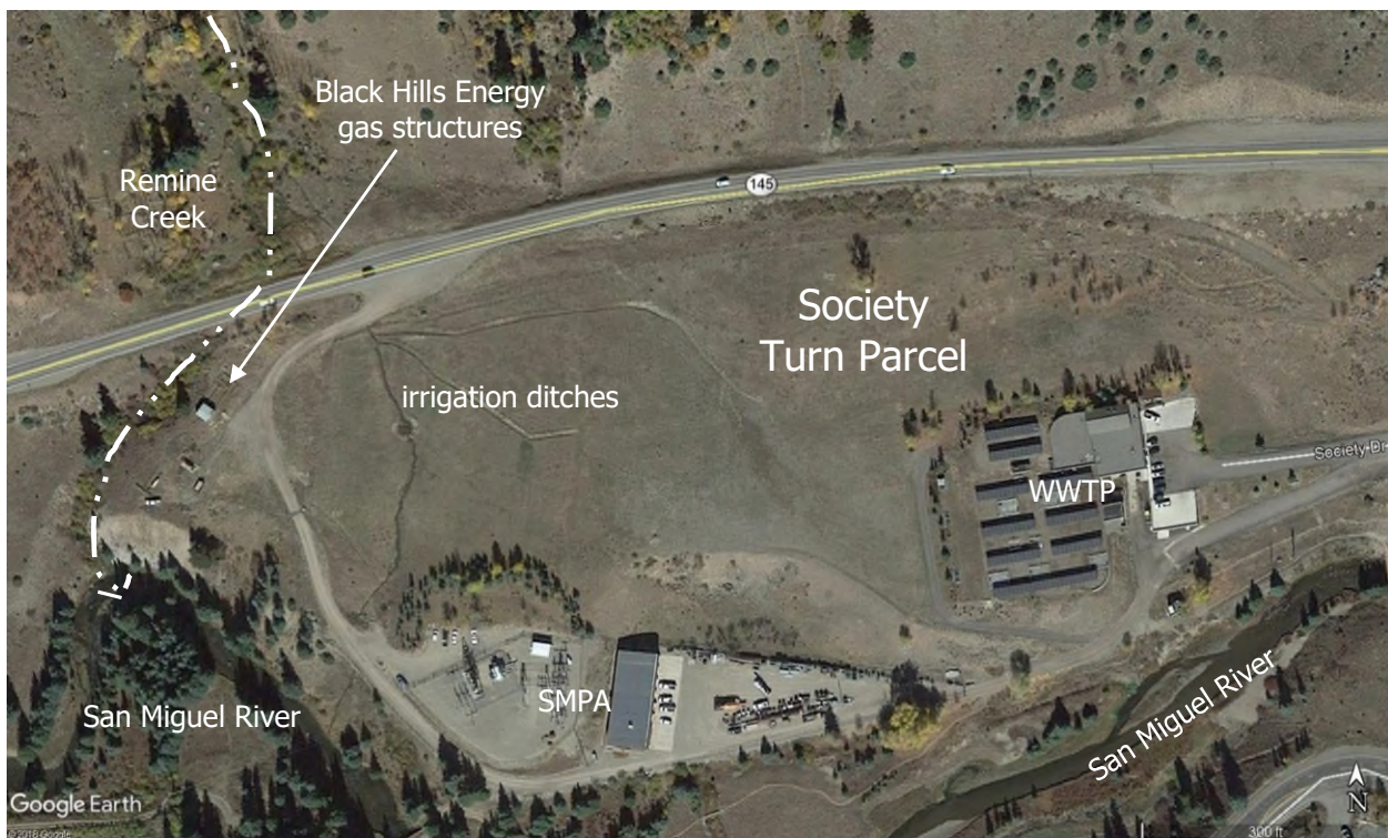
Photo 1. Aerial image of western portion of Society Turn Parcel. Note the location of the San Miguel River along the southern margin, the Remine Creek channel along the western portion of the Society Turn Parcel, and the three irrigation ditches in the western portion of the open field (Google Earth image, 10/12/15).
