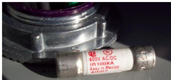
Figure 22 properly rated midget fuse (correct)
