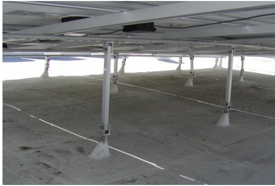
Figure 14 properly flashed roof penetration (correct)
