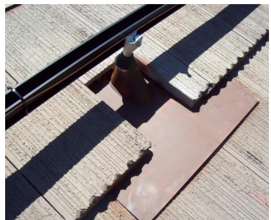
Figure 15 properly installed flashed roof penetration (correct)
