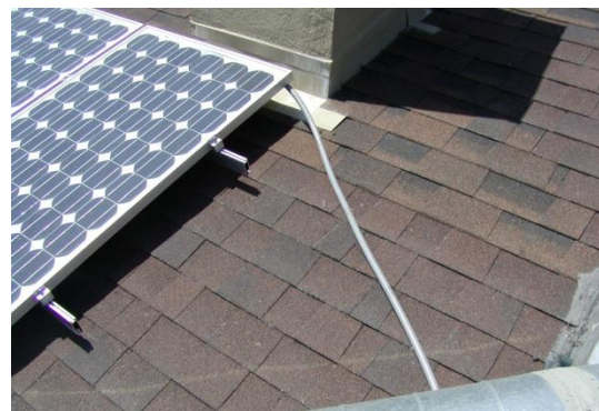
Figure 5 (incorrect) FNMC without support
