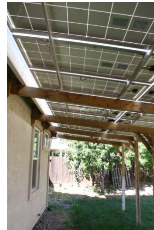
Figure 19 Wiring above 8 feet (correct)
