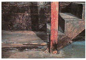
Figure 3.14. To prevent termite infestations, do not allow wood form boards to be embedded in concrete as shown in this basement.
