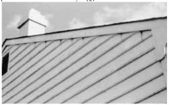
Figure 6.20. Carpenter bee damage.
