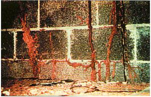
Figure 3.11. To reach wood in buildings, termite workers Often make mud tubes up the out side or inside of foundation walls. These tubes protect the workers from natural Enemies and help provide the moist environment they need.
