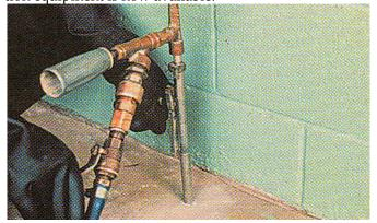
Figure 3.4 A slab injector used to inject termiticide under pressure into an area beneath a slab.
