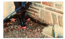
Figure 4.7. A typical basement treatment will also include trenching and rodding the outside perimeter of the foundation.
