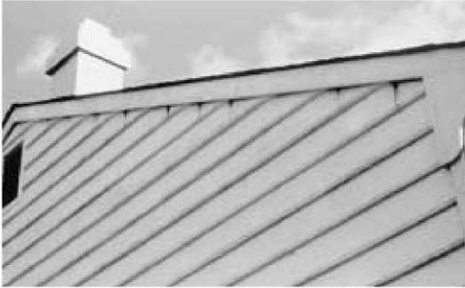
**Figure 6.20. Carpenter bee damage.**
