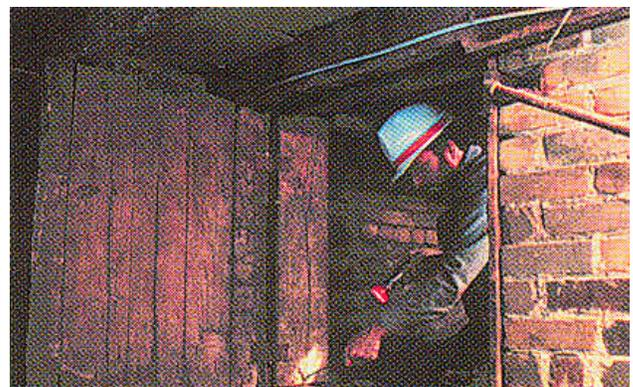
**Figure 3.9. Inspection of crawl space for termite infestations (he should also be wearing gloves).**
