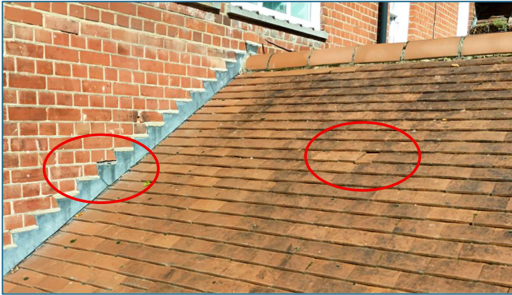
Example of missing mortar to lead stepped flashing, and a tile that has slipped.
