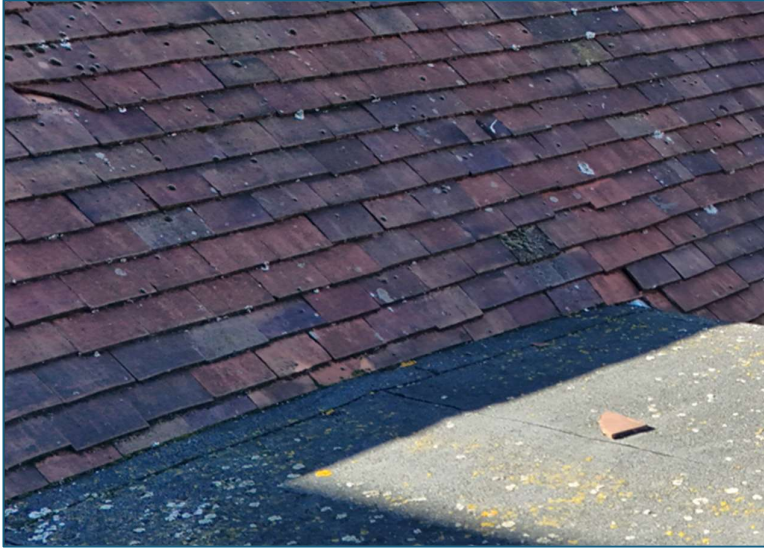
Example of where a broken tile has fallen onto the dormer roof below.
