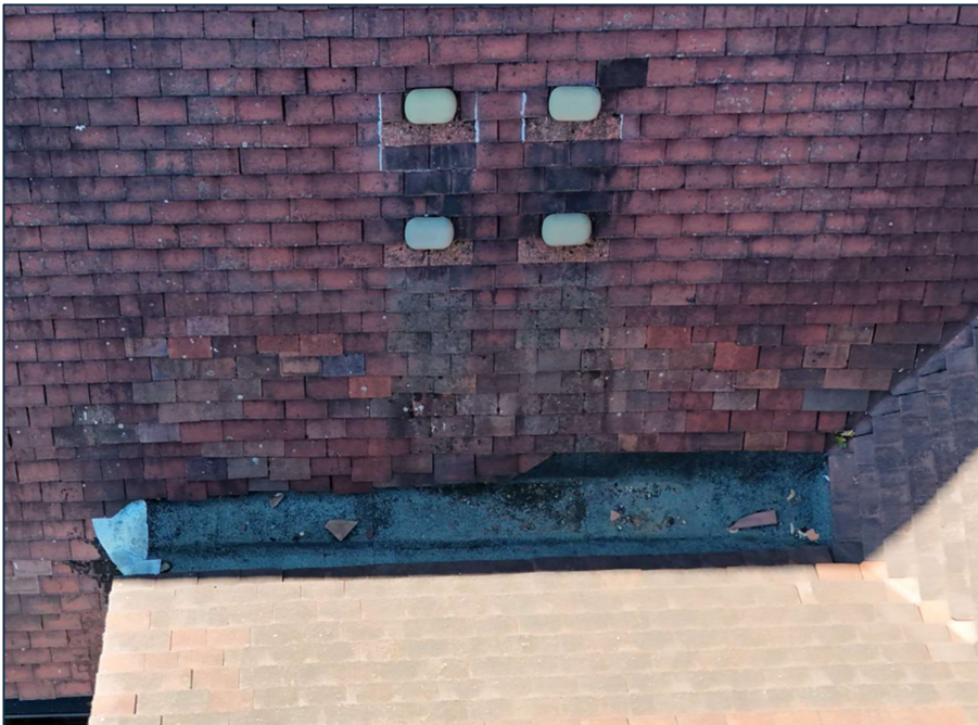
Further examples of slipped tiles.
