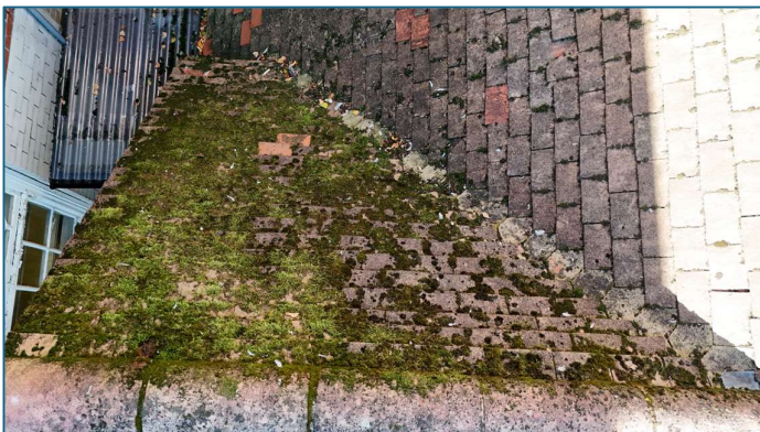
Moss/lichen build up visible. Evidence of previous tiles replacement.
