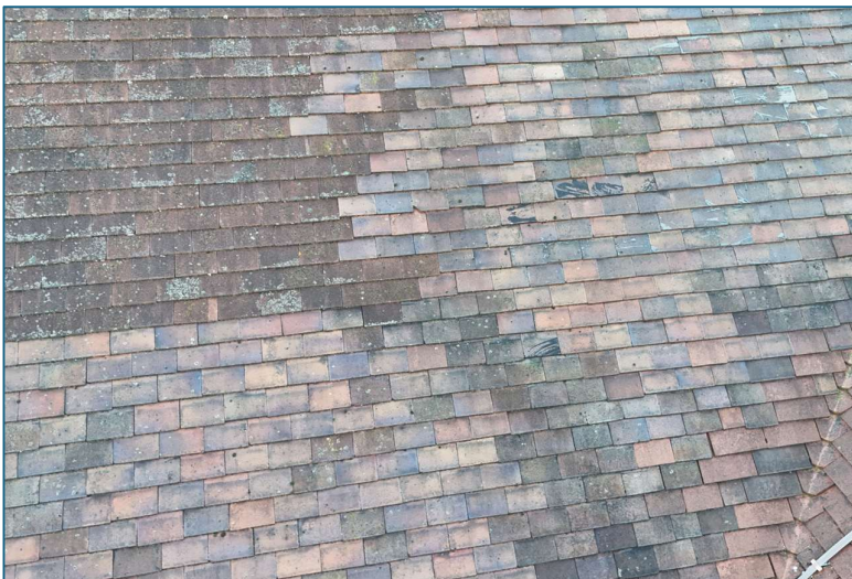
Various examples of defective tiles that are broken/slipped.
