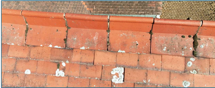
Example of eroded mortar between ridge tiles.
