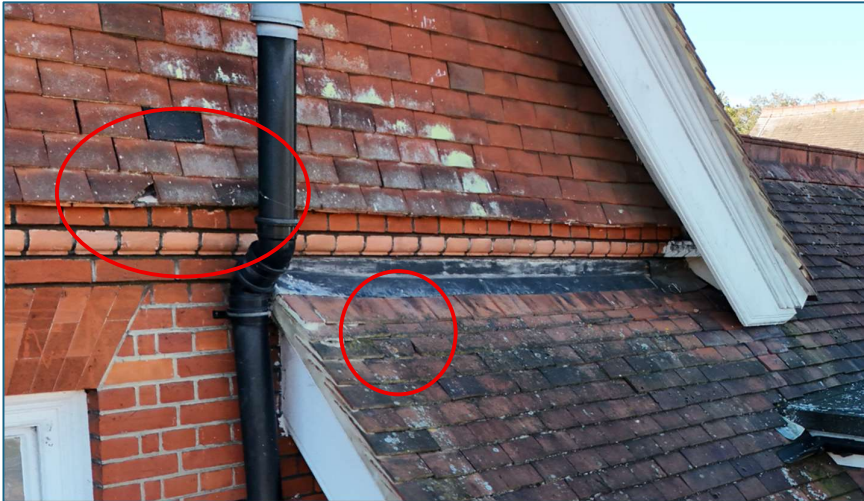
Example of broken tiles, leaving a possible route for water ingress.
