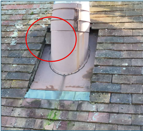
Example of tile that has dislodged.
