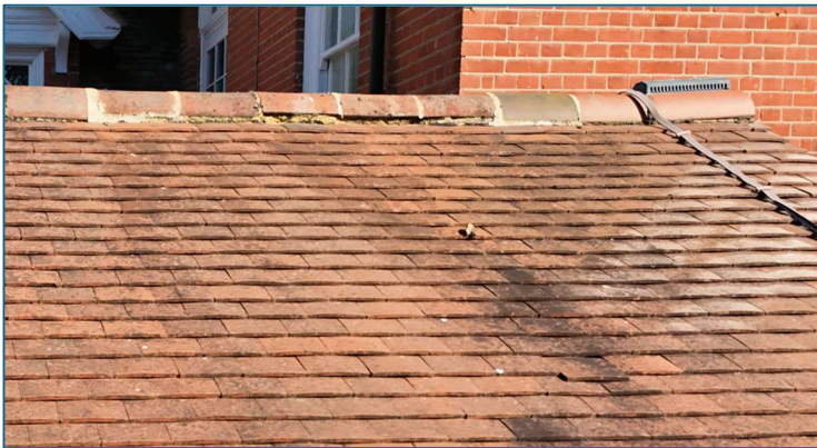
Mortar missing below ridge tiles, evidence of previous re-bedding of ridge tiles.
