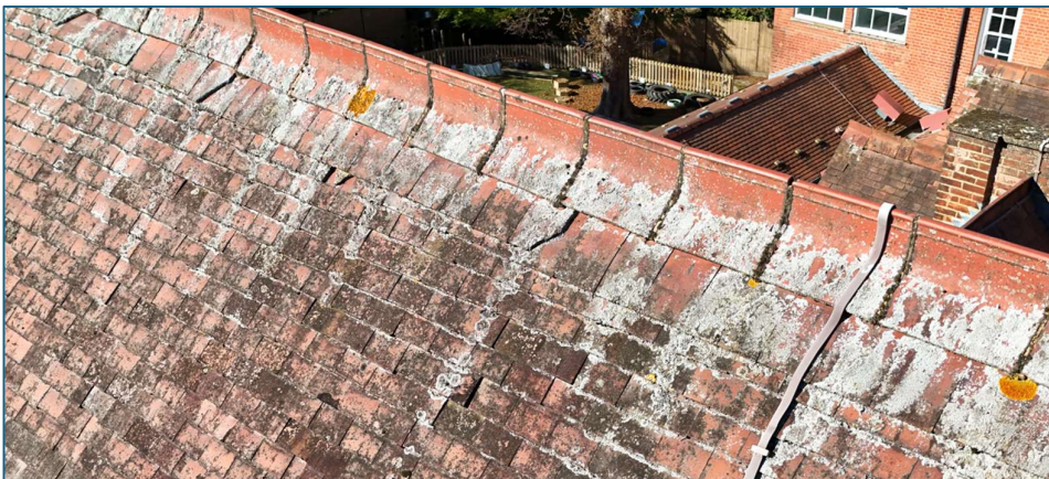
Example of broken tiles across the top row.
