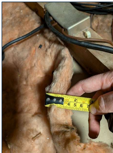
Photo 2 Existing mineral wool between joists
