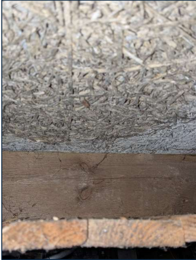
Photo 3. Underside of woodwool slab
