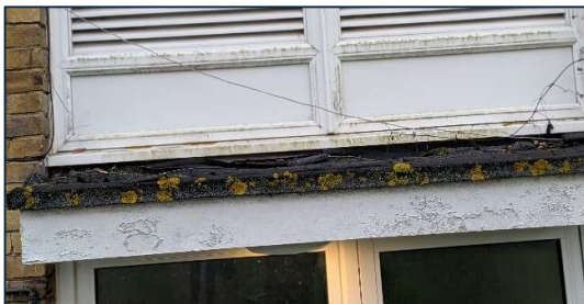
Photos 17: Canopy Roof – Typical Example
