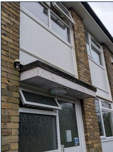
Photo 4. Typical Canopy Roof
