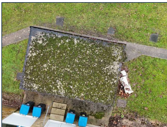
Photo 16: Aerial View of Bin Shed
