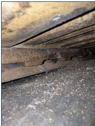
Photo 1. Underside of interlocking tiles
