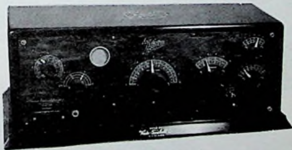
ZENITH 3R LONG DISTANCE RECEIVER 1923 4 TUBES $175.00
