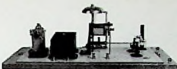
BRANLEY COHERER AND DECOHERER WITH KEY WIND TAPE PRINTER ABOUT 1902 TO 1905
