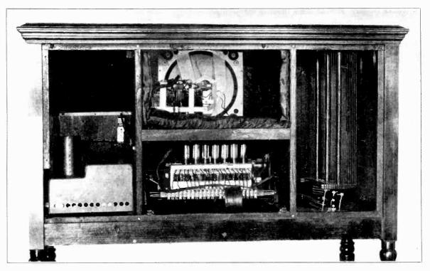
Figure 1-Back view of Radiola 30 showing arrangement of parts
