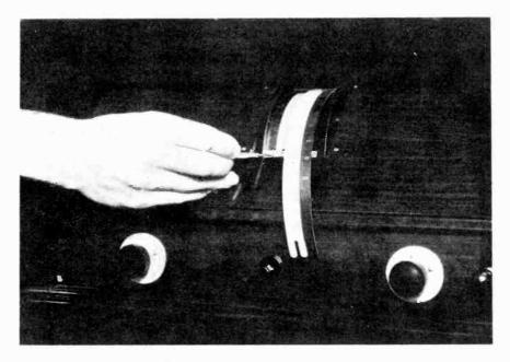
Figure 21-Replacing tuning drum dials
