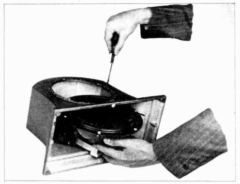
Figure 3—Removing mechanism assembly from housing
