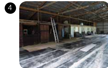
The barn has been converted into dorm rooms.
