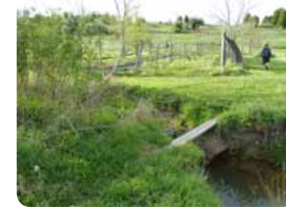
Flooding and lack of vegetation undercut the creek banks.
