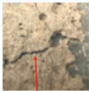
Specimen cracked intentionally
