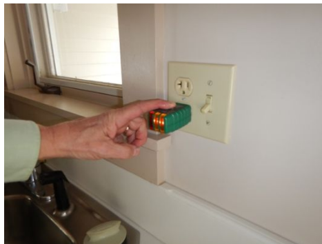
No GFCI protection
