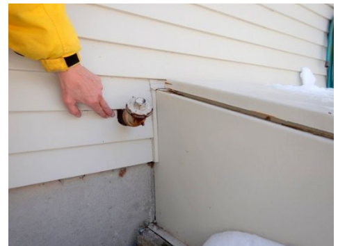
Missing sealant
