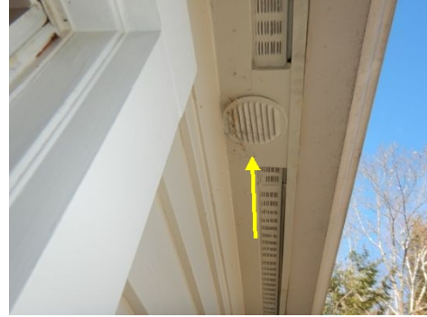
Tightly louvered duct
