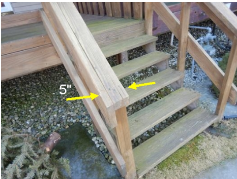
No graspable handrail
