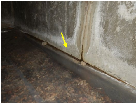
Seepage below crack
