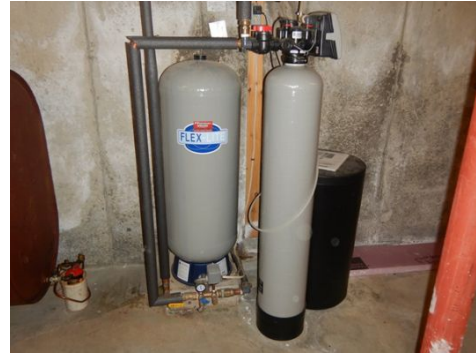
Basement well equipment
