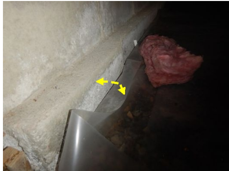
Vapor barrier not sealed
