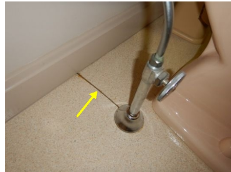
Lifting seam
