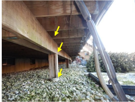
Direct weight bearing
