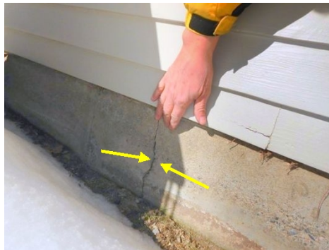
Unsealed crack
