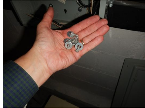
Sharp tipped cover screws
