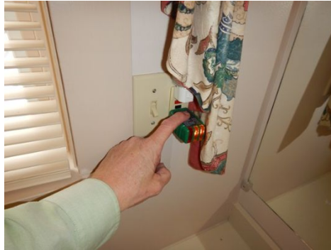
GFCI not responding
