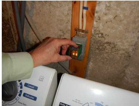
No GFCI protection
