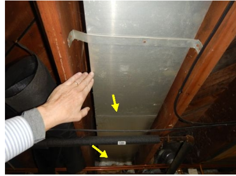
Unsealed duct joints
