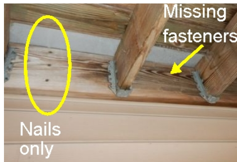
No structural connections; missing fasteners
