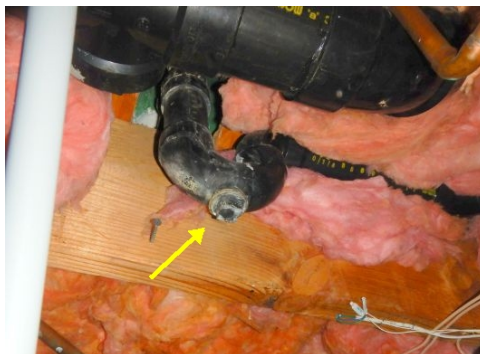
Leaking shower trap
