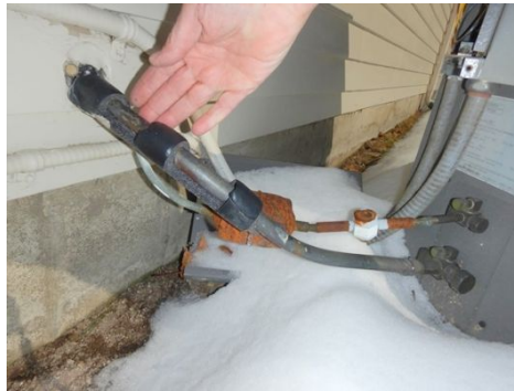
Worn insulation
