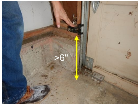
Excessive electric eye elevation
