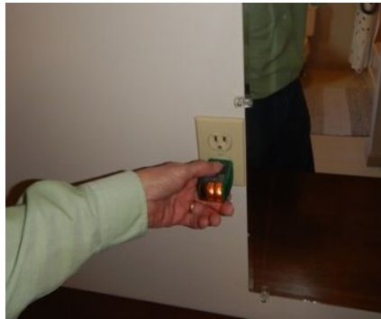
No GFCI protection
