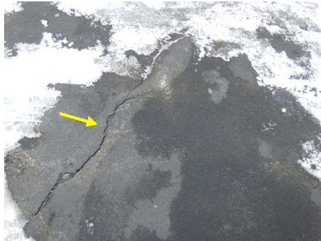
Opening cracks
