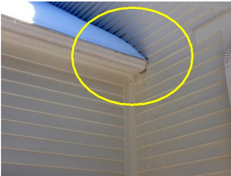
No kickout flashing
