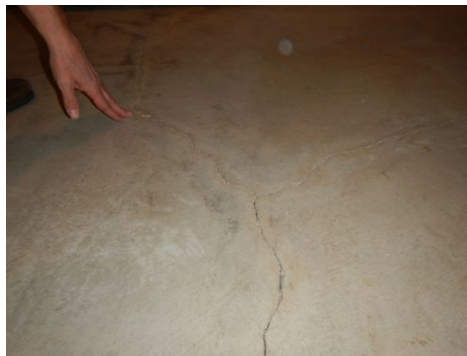
Unsealed cracks
