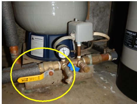
Water shut off
