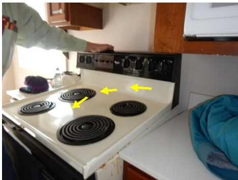
Missing tip protection
