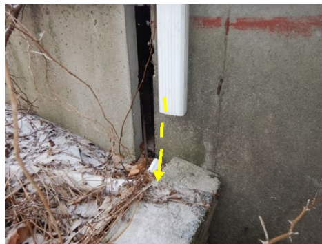
Discharging against foundation
