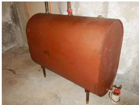
Basement oil tank
