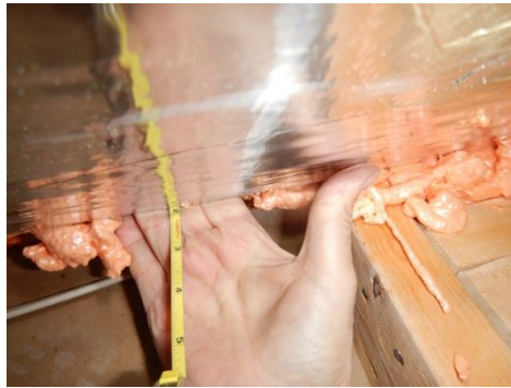
Front eaves insulation
