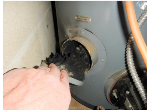
Loose inspection port plug
