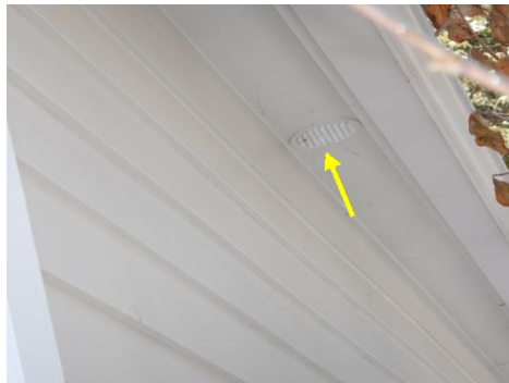
Tightly louvered vent
