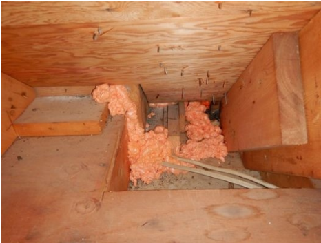
Air sealed penetration
