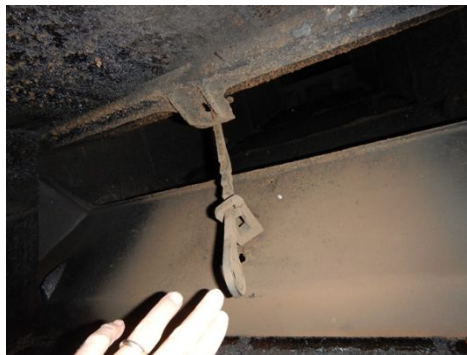
Damper out of alignment
