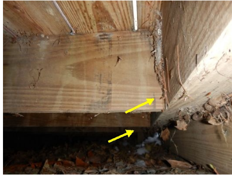
No joist hangers
