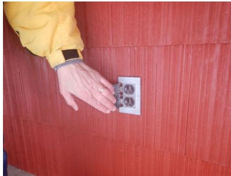
No GFCI protection
