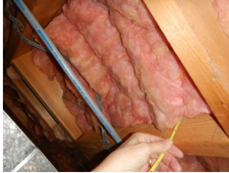
Floor joist insulation
