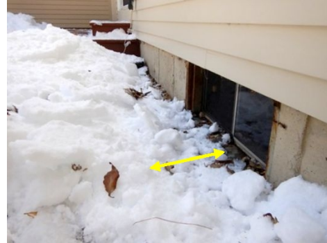
Even with basement windows
