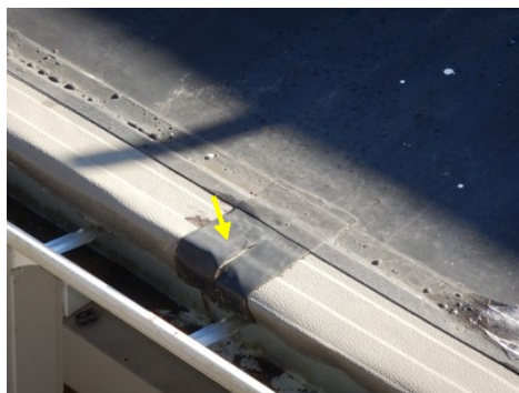
Opening seam on metal edge
