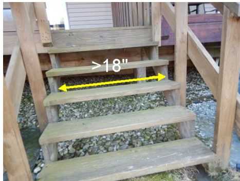
Widely spaced stringers
