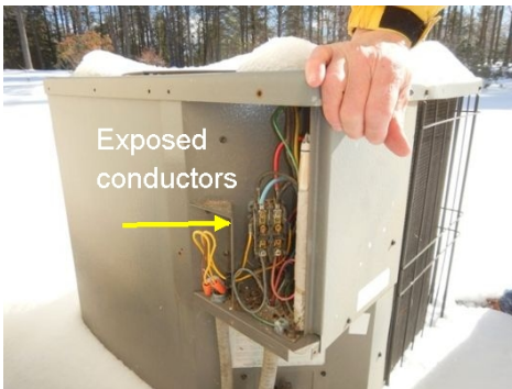
Missing cover panel
