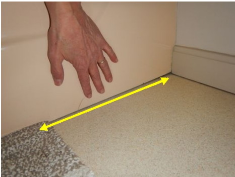
Not sealed against tub
