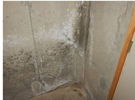
Efflorescence and dampness in corners
