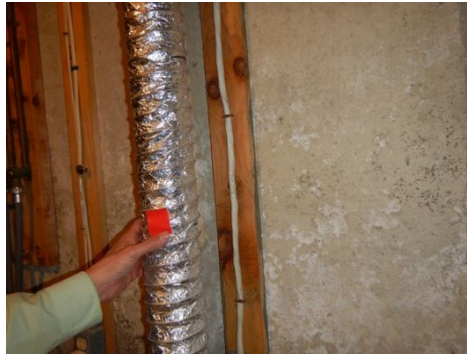
Flammable duct
