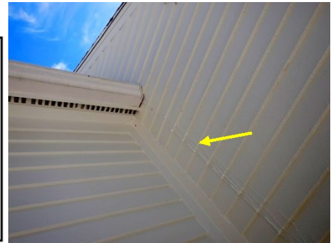
Water wash along siding
