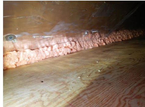
Visible air sealing
