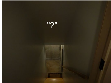
Minimal basement stair illumination
