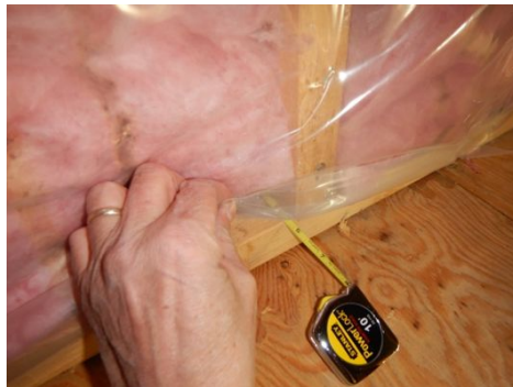
Visible wall insulation
