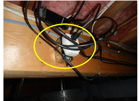
Missing cover plate
