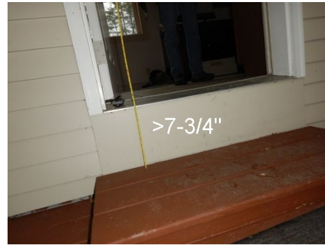
Excessive step height
