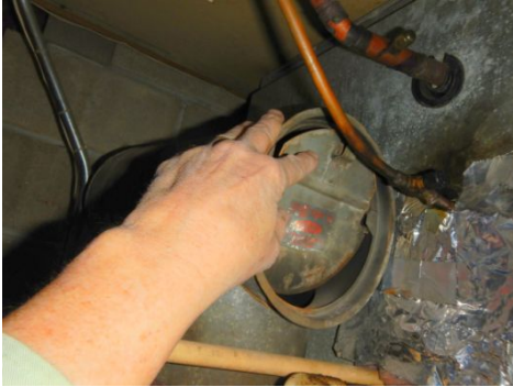
Missing damper counter weight
