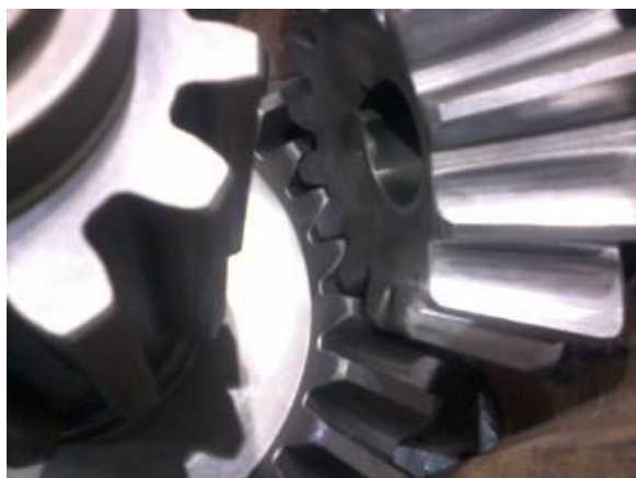
Checking gear backlash inside of an ST-80 gearbox
