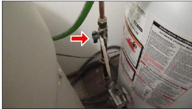
7.1 Item 2(Picture) Water heater gas shut off valve
