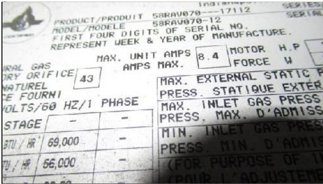
9.0 Item 5(Picture) Carrier furnace specification tag
