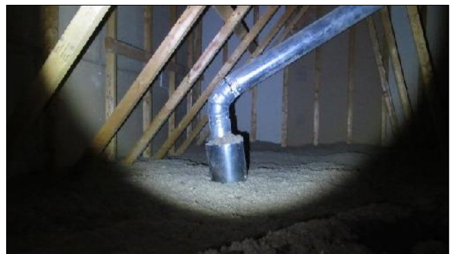
7.8 Item 2(Picture) Venter pipe through ceiling
