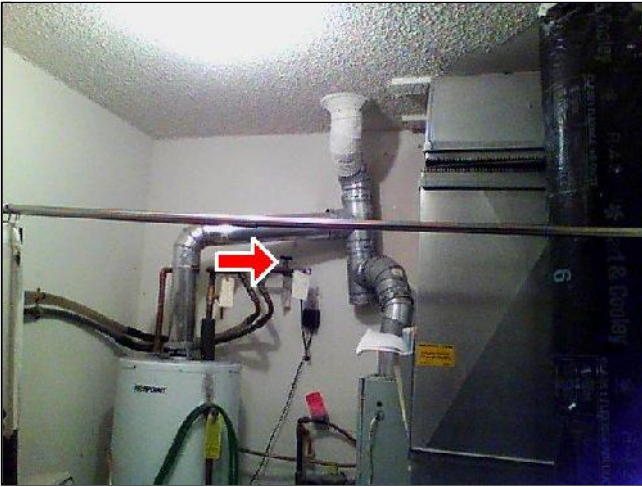
7.0 Item 1(Picture) Main water shut off
