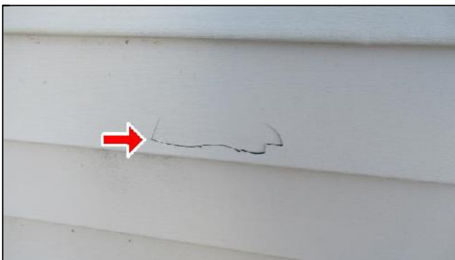
2.0 Item 3(Picture) Hole in siding
