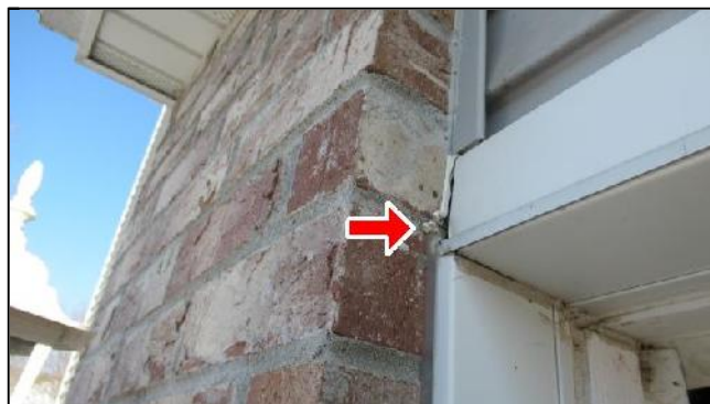
2.0 Item 4(Picture) Caulking on brick veneer and garage
