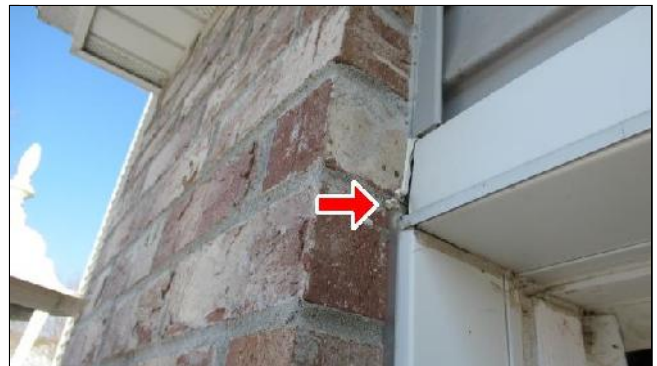
2.0 Item 4(Picture) Caulking on brick veneer and garage
