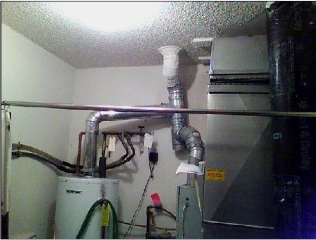
7.8 Item 1(Picture) Furnace and water heater vent system
