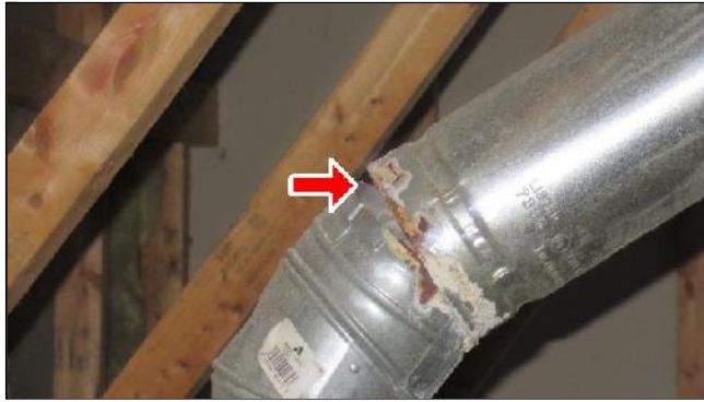
7.8 Item 3(Picture) Vent pipe elbow separation
