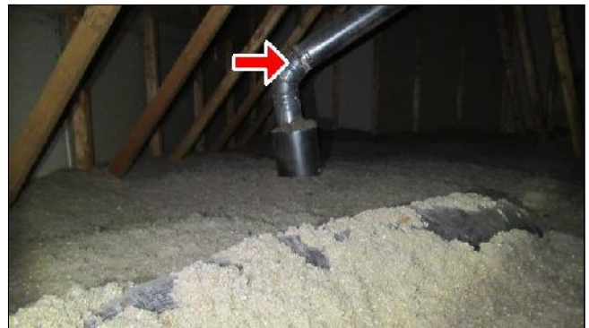
7.3 Item 2(Picture) Water heater exhaust vent
