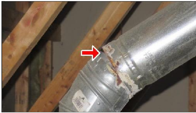
7.3 Item 3(Picture) Exhaust vent separation
