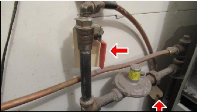
7.1 Item 1(Picture) Furnace gas shut off
