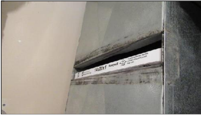
9.0 Item 3(Picture) Furnace filter location
