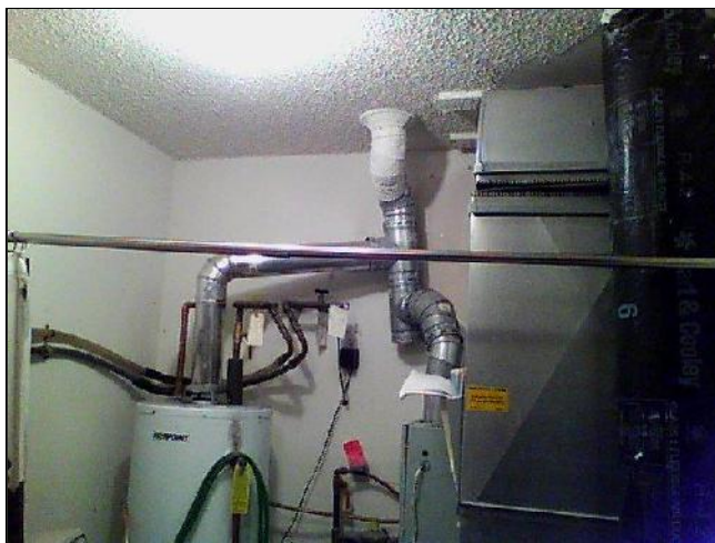
7.8 Item 1(Picture) Furnace and water heater vent system
