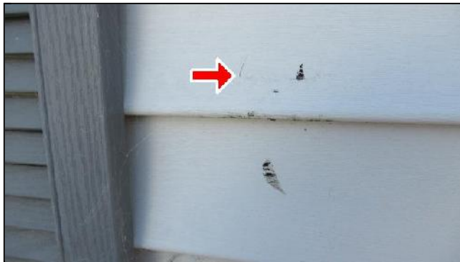
2.0 Item 1(Picture) Hole in siding
