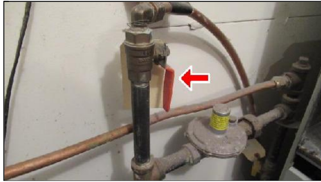
9.0 Item 4(Picture) Furnace shut off
