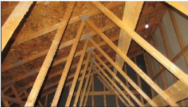
4.6 Item 1(Picture) Attic truss
