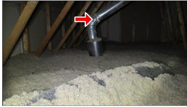
7.3 Item 2(Picture) Water heater exhaust vent
