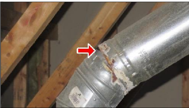
7.8 Item 3(Picture) Vent pipe elbow separation
