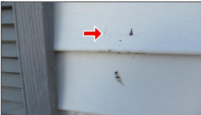
2.0 Item 1(Picture) Hole in siding
