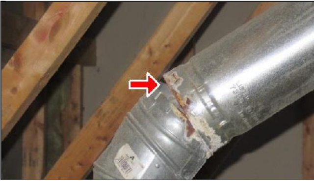
7.3 Item 3(Picture) Exhaust vent separation
