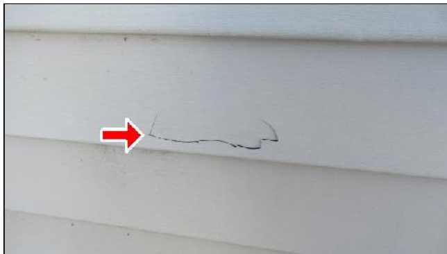
2.0 Item 3(Picture) Hole in siding
