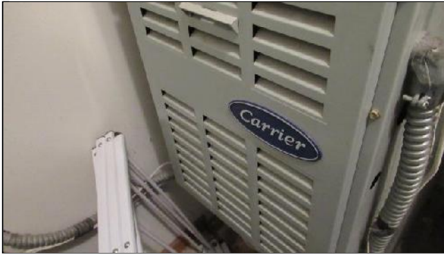
9.0 Item 1(Picture) Forced air gas furnace
