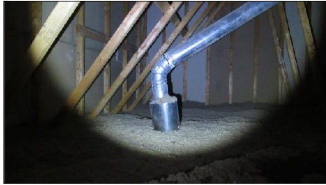
7.8 Item 2(Picture) Venter pipe through ceiling
