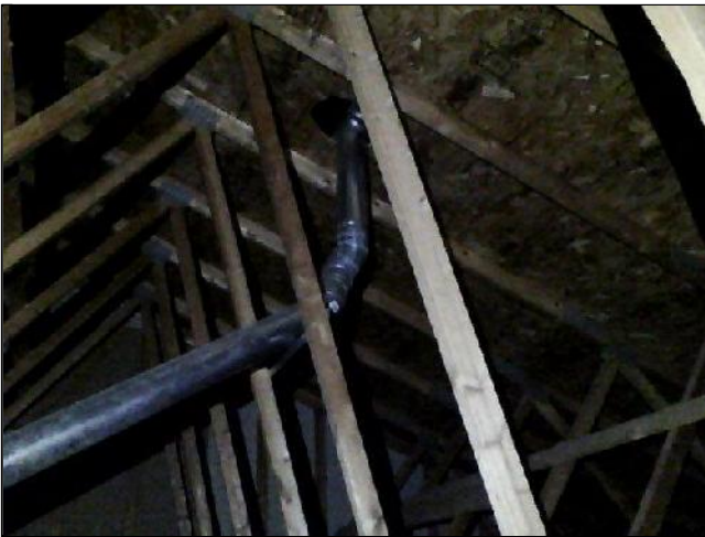
7.8 Item 5(Picture) Vent pipe through roof location
