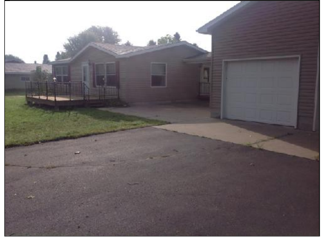
Side (facing west)
