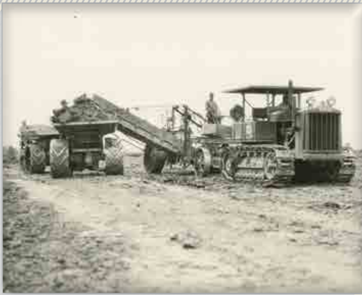
This Cletrac 100 is operating an elevating grader.
