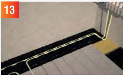
Complete the first circuit and connect the return pipe to the manifold using a euro cone connection. Repeat all circuits
