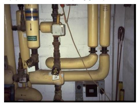
• Moulded or preformed lagging - generally used in thermal insulation of pipes and boilers. •
