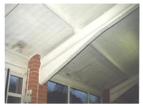
Sprayed asbestos - generally used as fire protection in ducts, firebreaks, panels, partitions, soffit boards, ceiling panels and around structural steel work.
