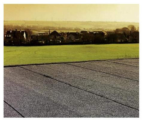
• Bitumen roofing material.
