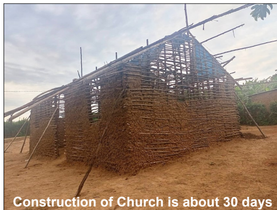
Construction of WAY Church
