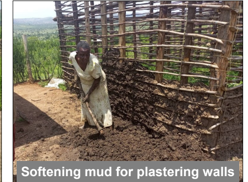
Digging soil to make into mud
